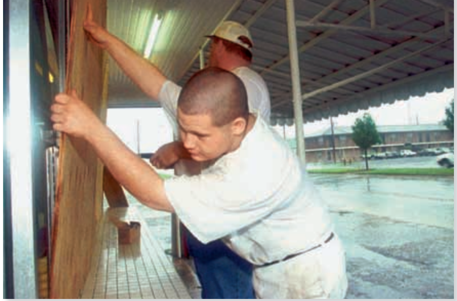
Figure 17 The people in this picture are preparing for a hurricane. The wooden boards help protect their windows from the high winds of a hurricane.
